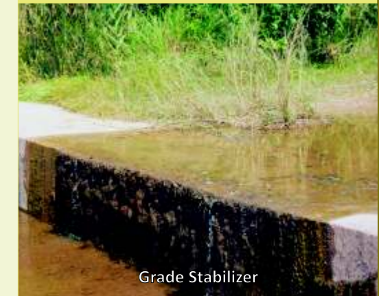
Gully plugging structure in Catchment Area
