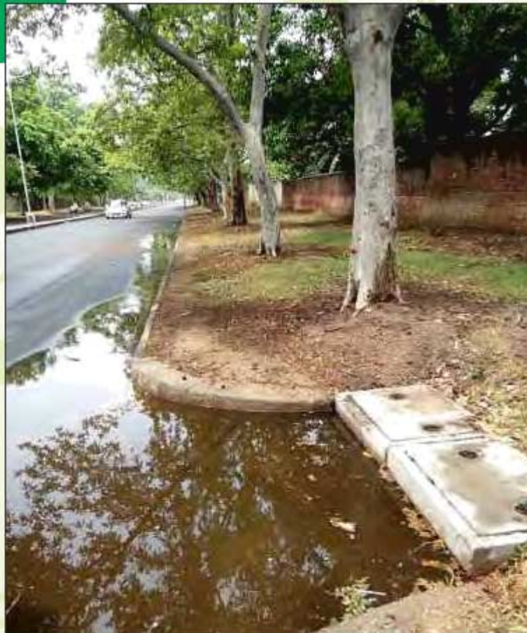
Picture 48: Sewerage blockade with Arjun seed capsules
